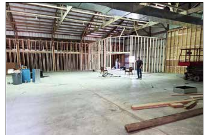
Construction is going on inside the main building at the Caring Hearts Campus.
