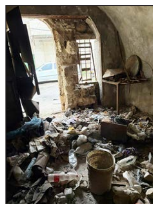
Before Hebron's restoration
